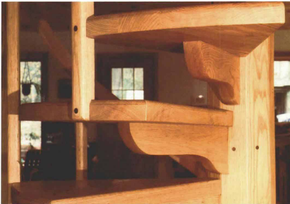
The treads and brackets were screwed and glued together, then bolted through the central post. Each baluster was screwed to two treads—mortised into the upper one and scribed over the lower. Photo by Wendy Jackson.
